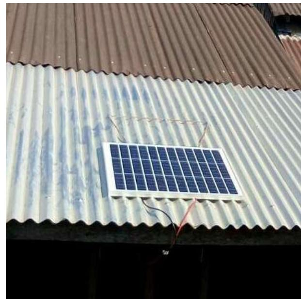
**Figure 4** Roof-mounted 50 W solar panel in Kyutawwa Village at Thongwa Township
